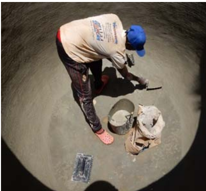
Figure 18.5 Finishing inside a calabash cistern. (Source: Author's own).
