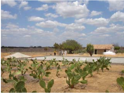
Figure 16.6 Cistern of 52,000 L with catchment area for irrigation of fruit trees and vegetables, near the house a cistern of 16,000 L with drinking water. (Source: Author).
