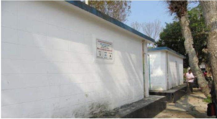
Figure 7.10 CHB tank of Morrelganji Health Complex. (Source: Author's own).
