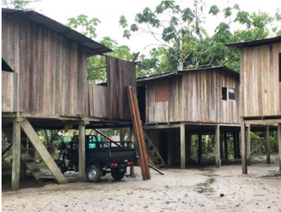
Figure 6.3 Amphibian houses adapted to rainfall and flooding in Putumayo, Amazonia. (Source: Author's own).
