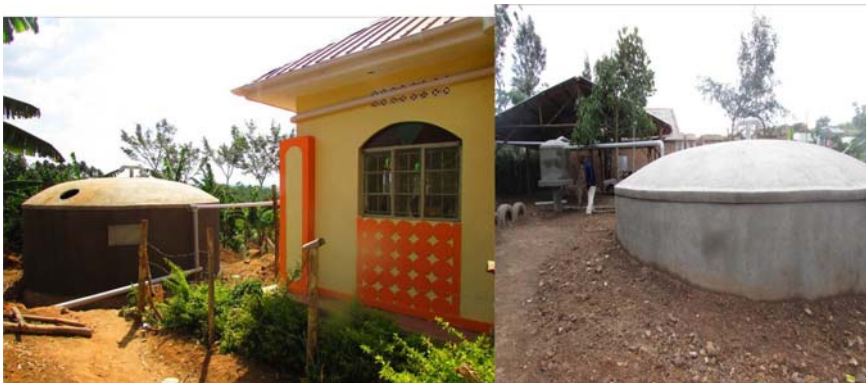
Figure 9.1 50 m 3 ferrocement tanks. (Source: Kikundwa Anne).
