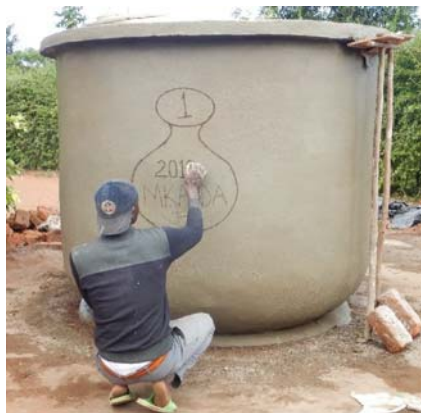
Figure 18.6 Finishing the outside. (Source: Author's own).
